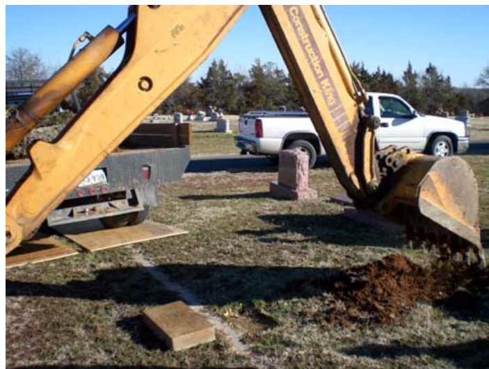
Photo No. 2: Excavation begins of the subject grave site on February 19, 2007.
