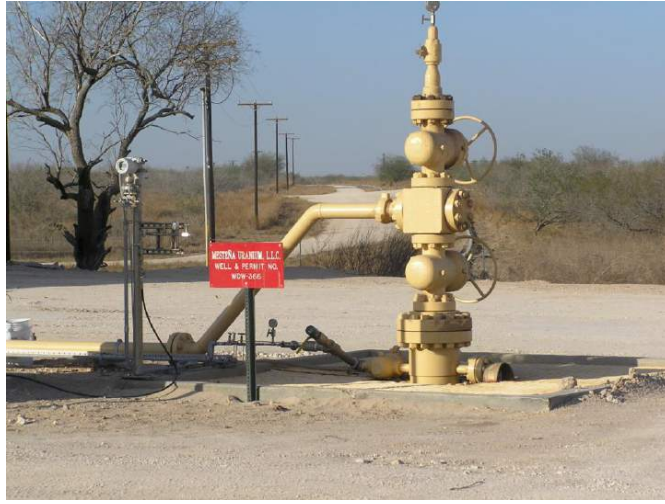
Figure 29 – One of MULLC’s Waste Injection Wells.
