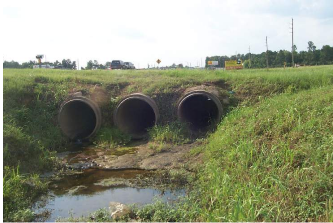
Figure 53 – GPR Depth Calibration Site. Looking North along Highway 249, South of Tomball, Texas (Near GPR Profile 4. See Figure 61, Profile 4c)
