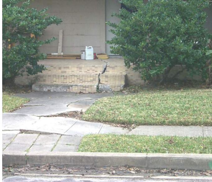
Figure 67 – GPR Profile 5: Hazard Street House (as of 2003) North to Right. Looking West (House Demolished in 2005 and Rebuilt)
