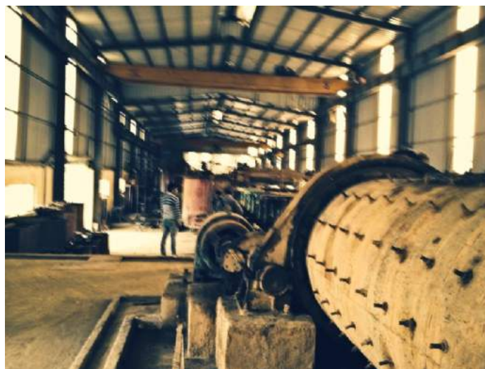
Figure 65 – Primary Crusher at the Processing Plant
