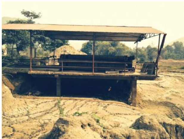
Figure 67 – Final Filtration System at Tailing Pond (Dry)
