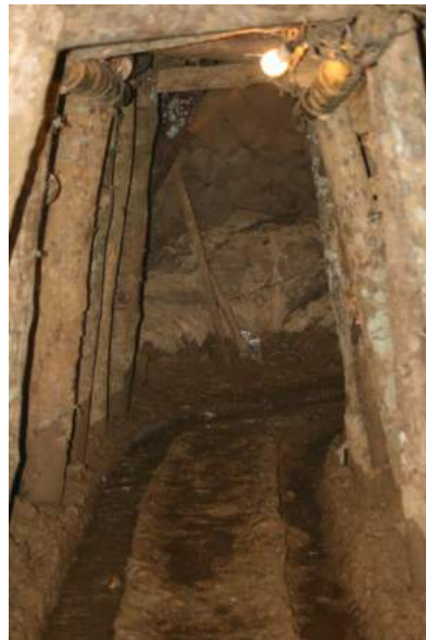
Figure 12 – Inside Hop Hoa Adit
