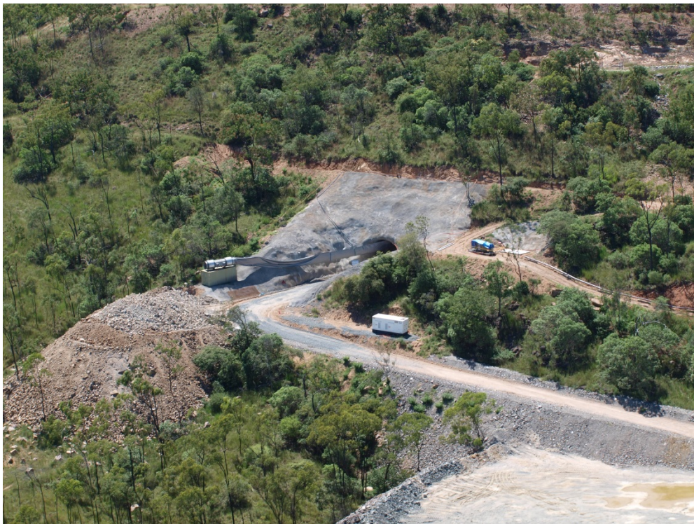
Mount Wright Mine (Haul Road at one of two Portals of Underground Mine) (see Figure 15 for Reference)
