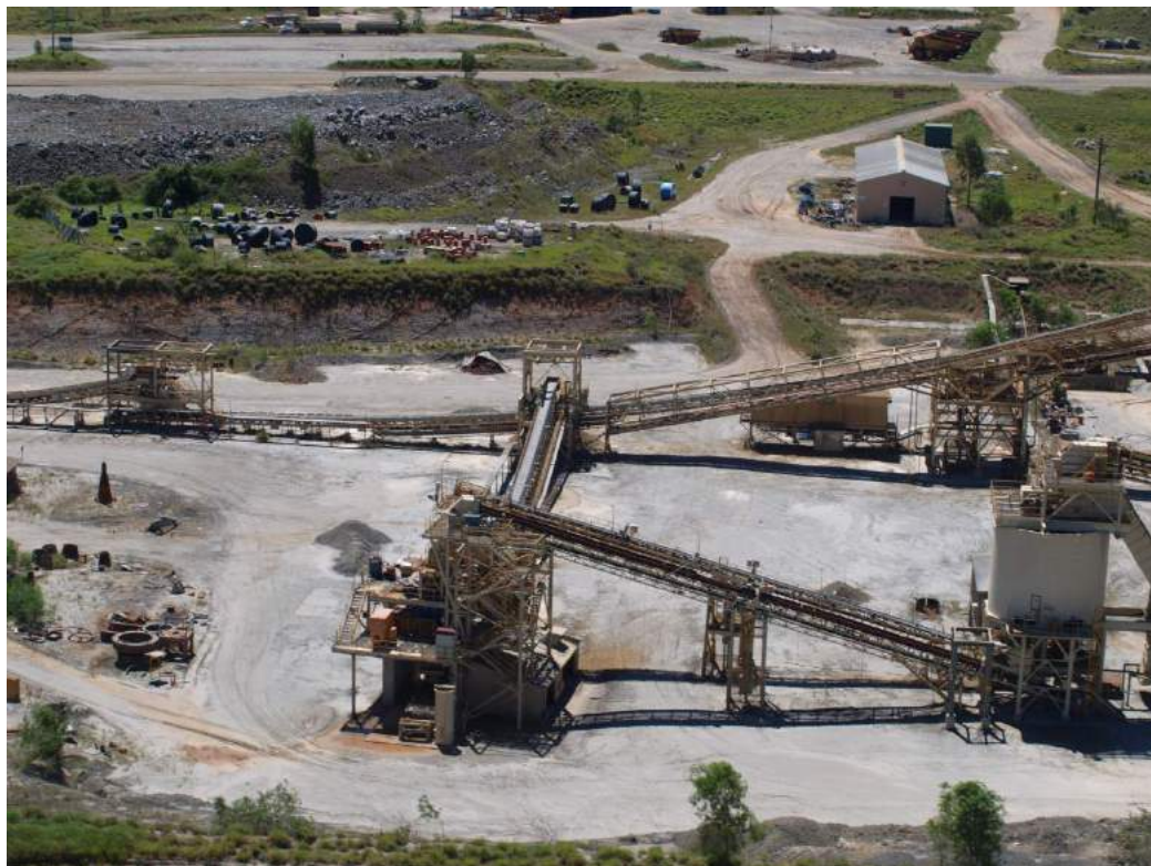
Primary Crushing Unit (to Handle Ore from Mount Wright Mine)
