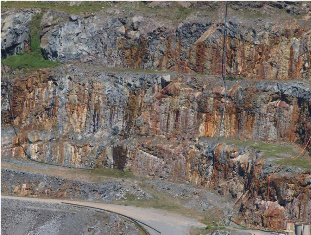
Views of Ravenswood Pit Walls – Pit Now Filling with Surface and Ground Water
