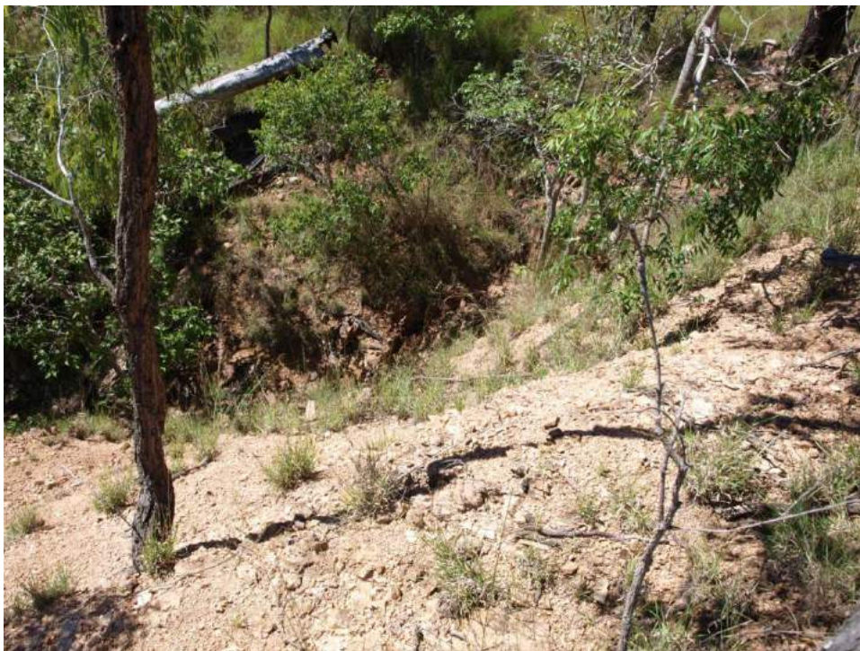
Central Area of Interest (Fault Contact between Two Units - light and dark-colored Units Likely at Fault Boundary between Units PCm and Ogpc of Figure 22)
