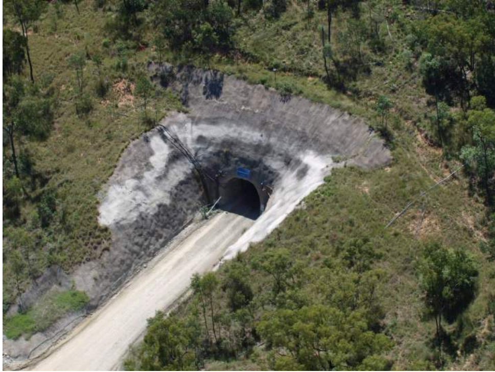
Mount Wright Mine (Second Portal to Underground Mine) (see Figure 15 for Reference)
