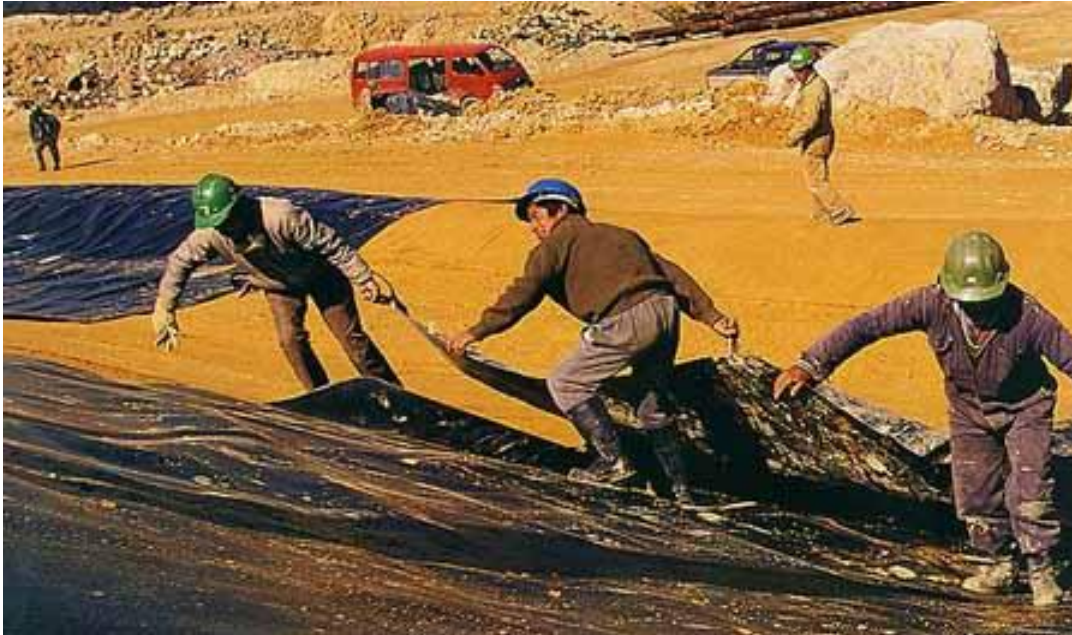
Installing a Plastic Membrane Liner
