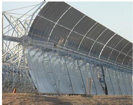
Parabolic trough at a plant near Harper Lake, California
