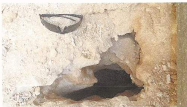
Figure 14. A void was encountered where the NP anomaly B is observed (see Figure 11). This void is enlarged to the north towards the McNeill High School and became a cave (Cave 5).
