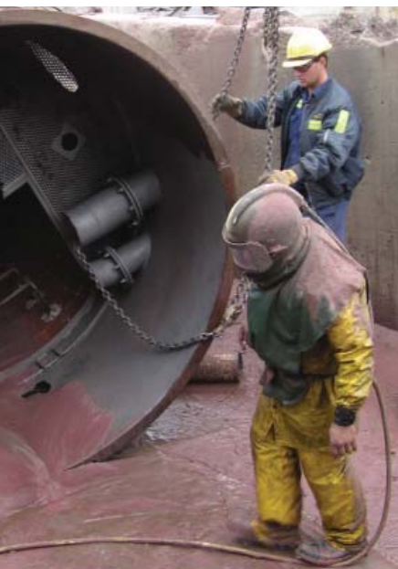
Cleaning NORM scale from coal washery vessels
