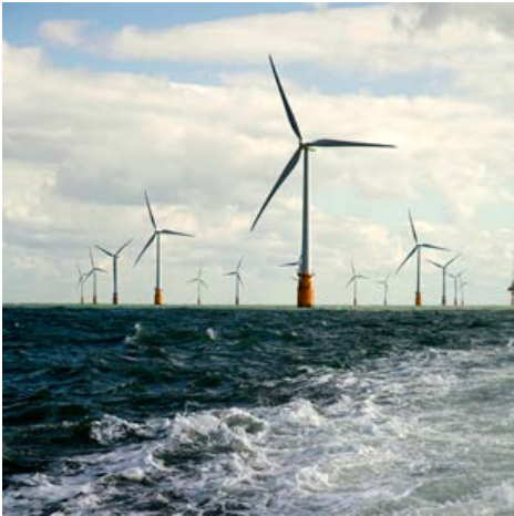
A wind farm off the coast of Britain that can generate 300 megawatts of electricity.
