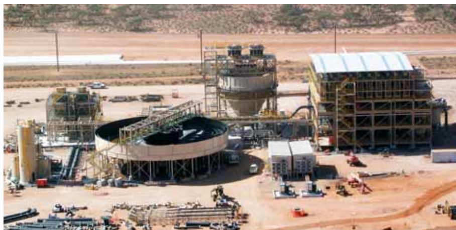
Figure 3 Wet concentrator plant — this was relocated from Iluka's operations in the United States. (Courtesy of Iluka Resources; photo 407879)
