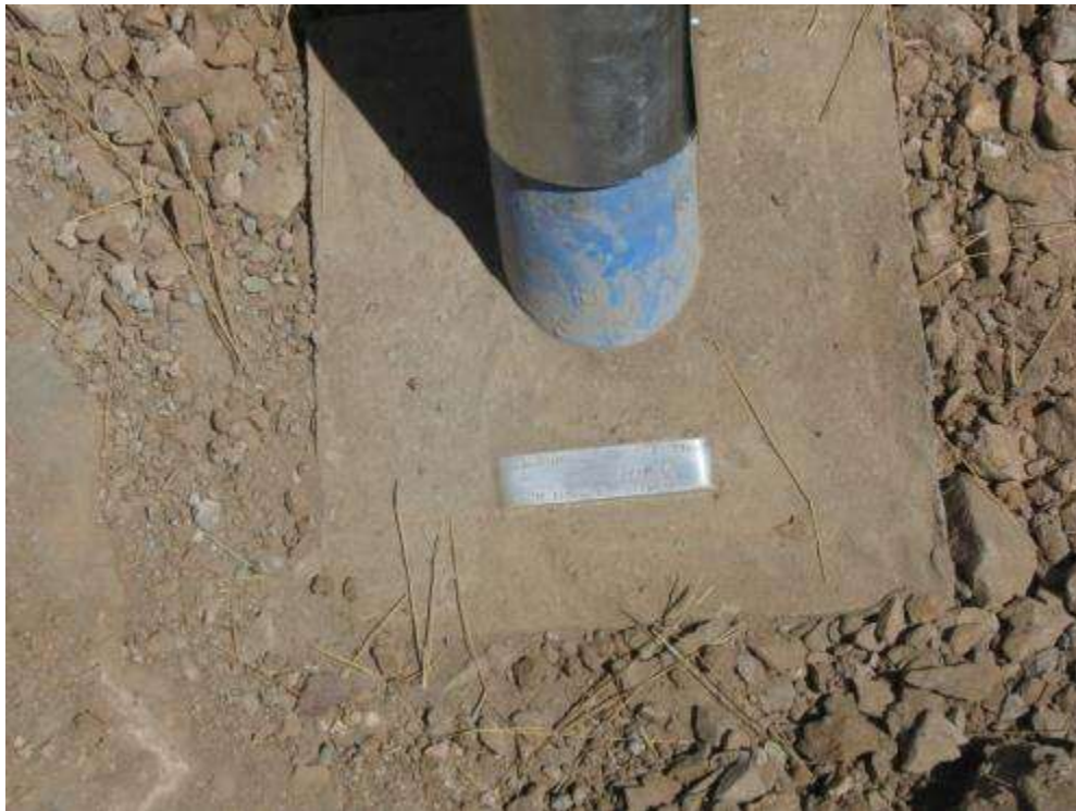
Plate 13.2 Completed borehole showing concrete plinth, marker and cover.
