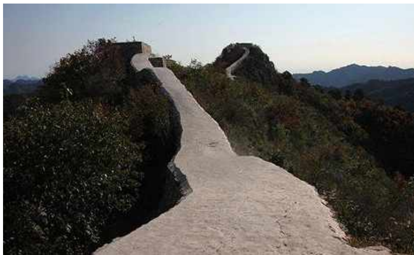
Figure 4.7 The Great Wall of Zhuizi mountain in the south of Xiaohekou Village, Yuzhong County, Liaoning Province(graphic source network)
