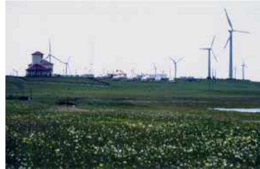
Figure2.14 Huitengxile Wind Power Plant(photo by the author)
