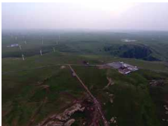
Figure 3.3 Wind power construction destroyed the grassland (photo by others)
