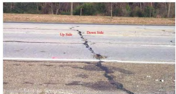
Figure 64: Recent Crack along GPR Profile 4: Willow Creek Area. Likely Caused by Dislocations Shown in Figure 62 as Profile 4b. Looking East across the Highway.
