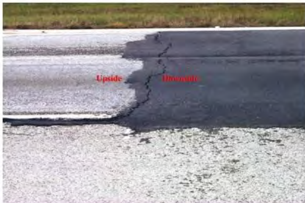
Figure 55: GPR Profile 1: Iowa Colony Site Looking West across the Northbound Lane (2005) (Note recent patch with more recent crack).
