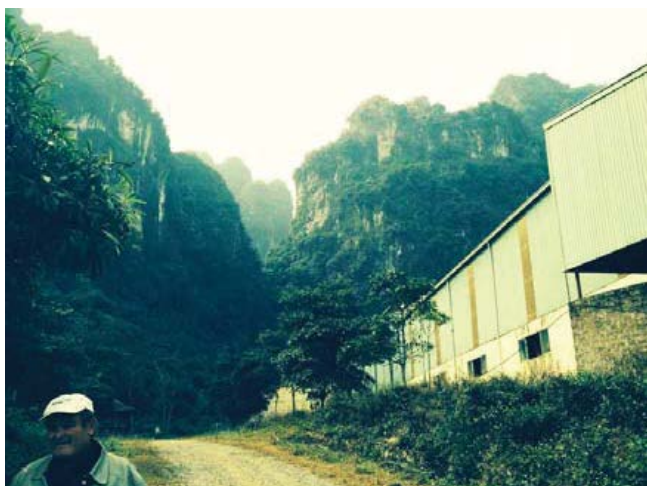
Figure 76: At the Processing Plant.
