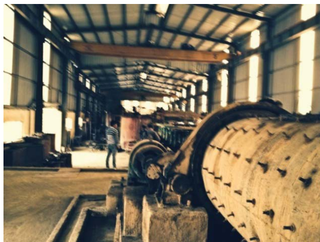
Figure 77: Primary Crusher in the Processing Plant.
