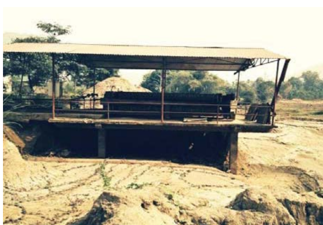
Figure 79: Final Filtration System at Tailing Pond (Dry).
