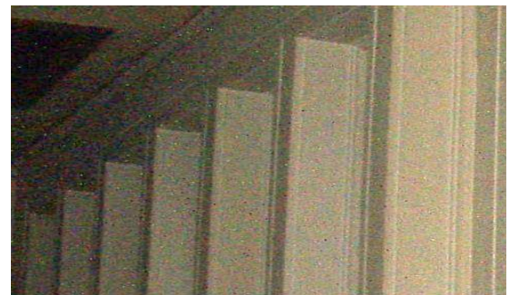
FIG. I.10. Photography of the buttresses (concrete beams) of the ceiling on the 4th floor of Building B of the Faculty of Physics (measured with GPR on Figure 1, 9). The same object is presented in Figure 1, 2, 9. Photo by Y.Shopov (Lab.Archeo-geophysics)
