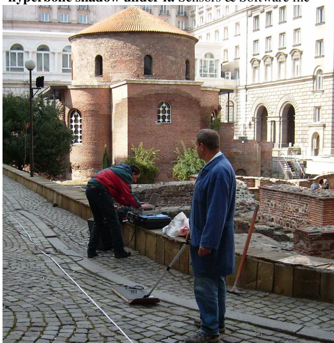
Fig. I.18. Scanning urban terrain with GPR for search of sewerage pipes by a team of archaeo-geophysics laboratory.
