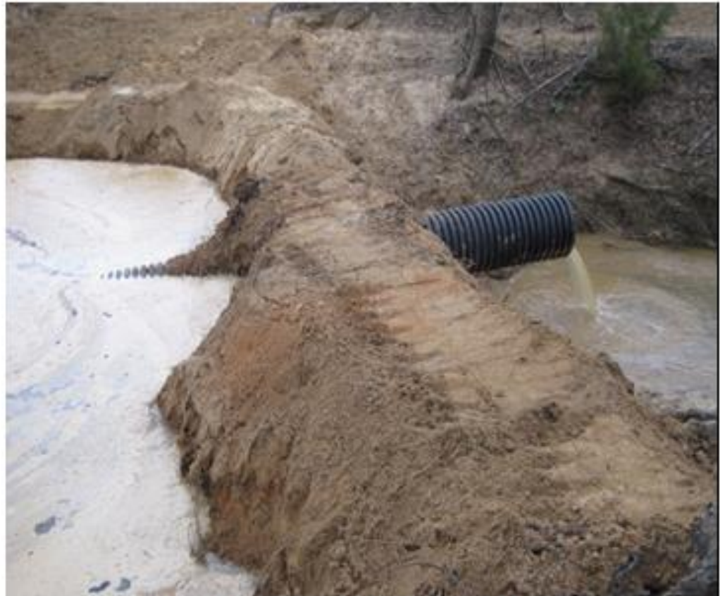
Finished emergency flume dam # 3.
