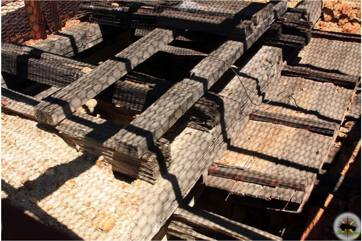
Figure 15. Bat grate over shaft at Morning Star Mine. From Destinations4x4.net (2020). Accessed Sept. 13, 2022.
