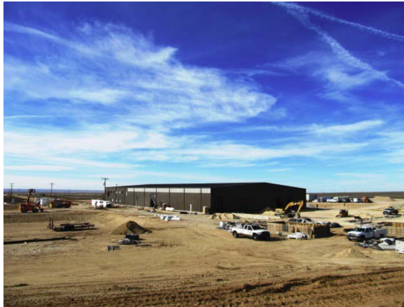
Figure 5 - UR-Energy's Lost Creek Plant Building 2012-13. Wyoming. (from Robert Odell)
