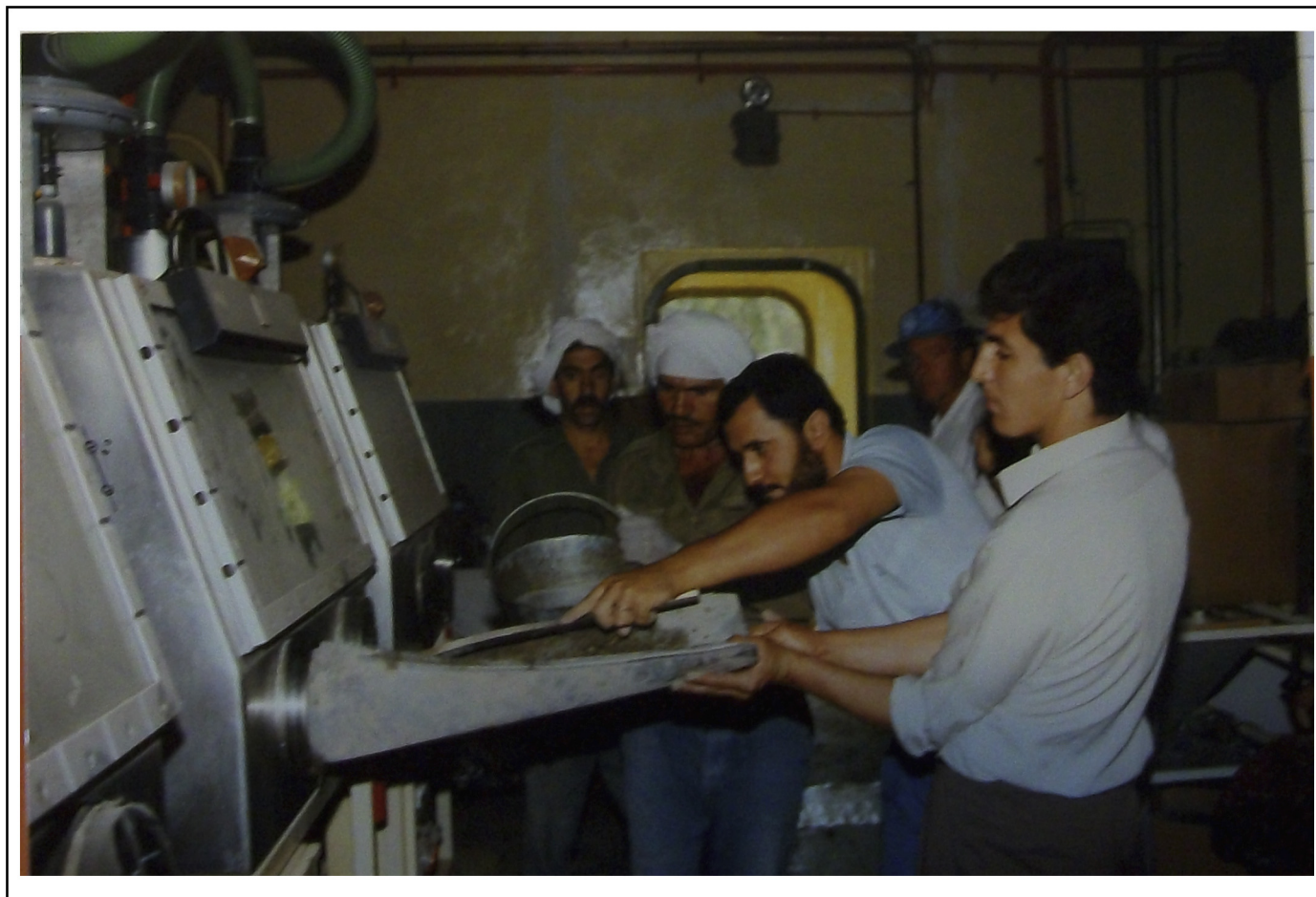
Figure 3. Under supervision of the IAEA team, Iraqi workers pour concrete into glove boxes so they can no longer be used for proscribed activities at Tuwaitha, October 1991, 7th United Nations inspection in Iraq. (Courtesy of the Archives of the International Atomic Energy Agency, no. 4954).
