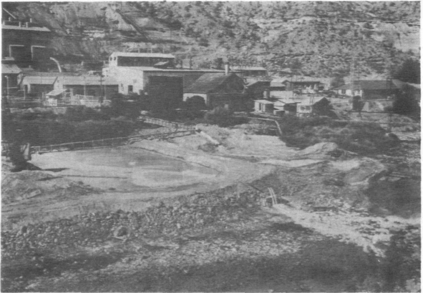
Organic-bearing raffinate is stored in ponds of this type. Because of its toxicity to aquatic life, this material should be disposed of by seepage or treated prior to discharge.
