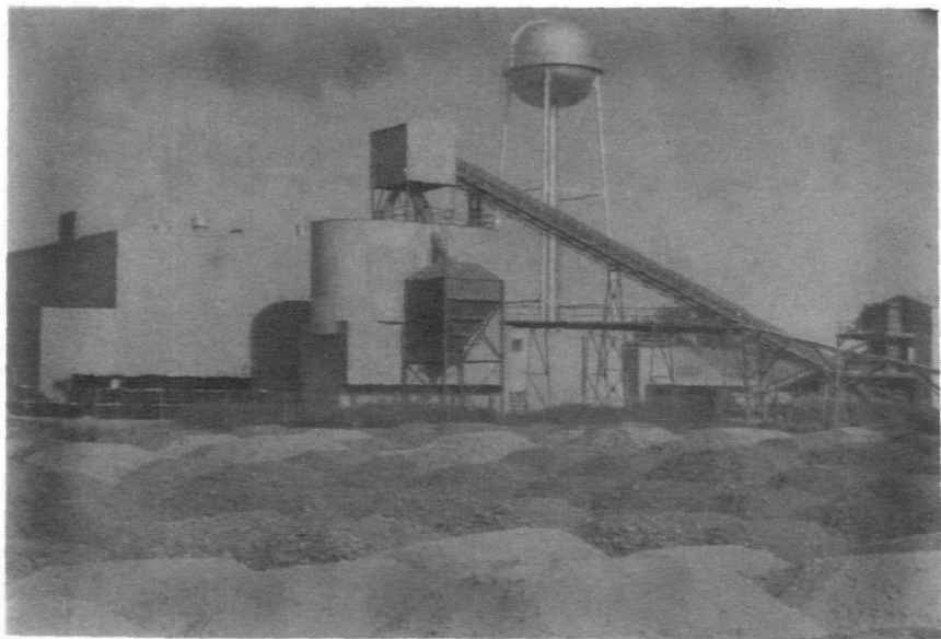
The ore is stored in separate piles according to uranium content. The various grade ores are blended prior to processing in order to stabilize the input to the mill. (Photograph courtesy of Mines development, Inc.)
